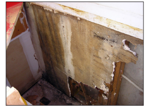
A slow leak caused mold to grow behind this counter. After a plumber fixed the leaky pipes, we came to remediate the mold.
